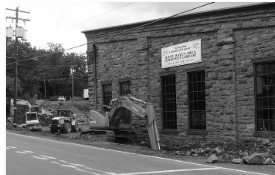
Digging the new drainage ditch along the west wall.
