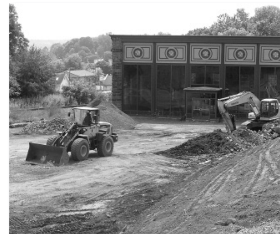
Grading the north end in preparation for the new parking area.
